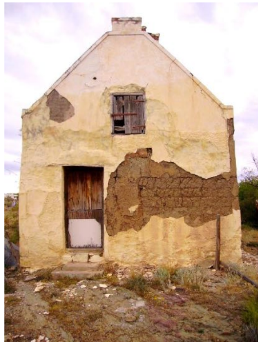
Photo 1: Layered appearance of the opgekleide walls at the old longhouse at Damascus. Gable end shows plaster band and traditional mock chimney cap (the chimney is concealed behind it).
